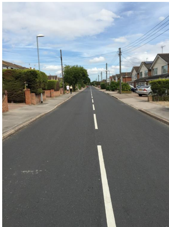
Facing east – highlighting the extent of vehicle crossings throughout.
