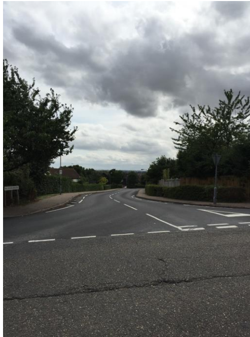
Facing south – looking into King Edward’s Road from Hamberts Road showing carriageway narrowing
