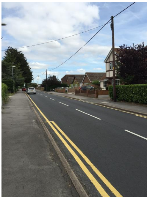
Facing east – showing existing parking restrictions
