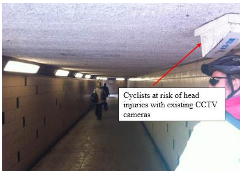
Photo 1 showing CCTV camera
