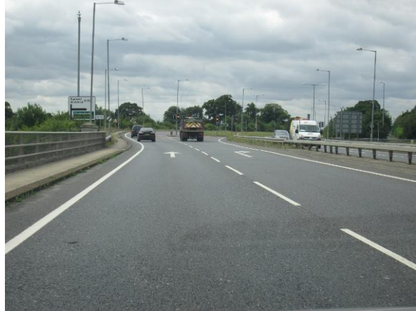
Image 2 – A132 SW bound approach to traffic signals
