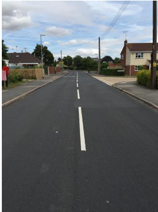
Facing east – towards the eastern end of King Edward’s Road showing access for adjoining roads
