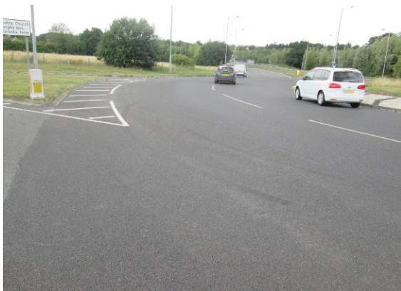
Image 3 – A131 NB road users straddling the roundabout circulatory markings
